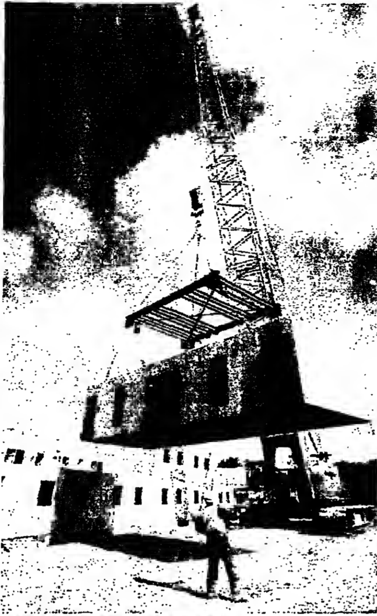
Precast units being craned into position at Fazakerley
